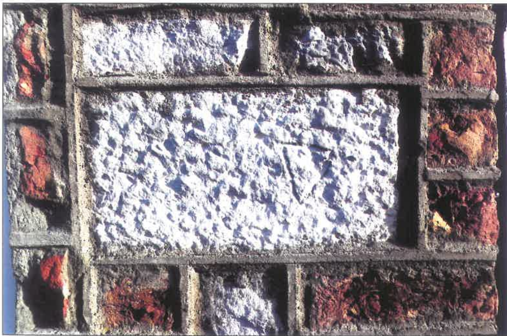
Fig. 2 Cat. No. 2 Masons' Mark on a reused stone in the Abbey Street Facade of Seodín Eile.
