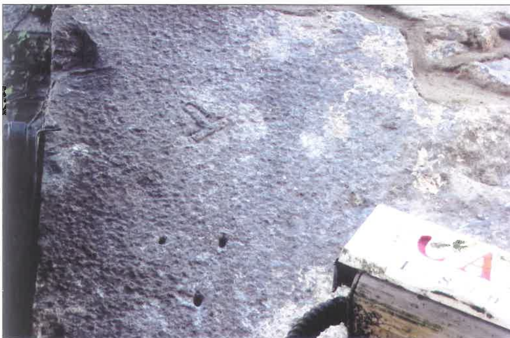
Fig. 3 Cat. No. 3 Medieval ashlar block reused as a quoin stone on the surviving part of the house of John Cruce of 1658, now part of Cruise's Hotel.
